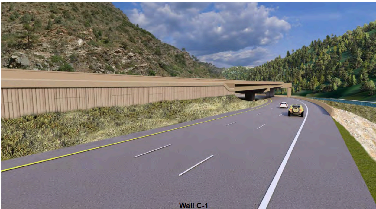
Wall C-1 looking east on EB with Bridge M and WB 1-70 in view. The wall is seen here with 5x10 panels.
