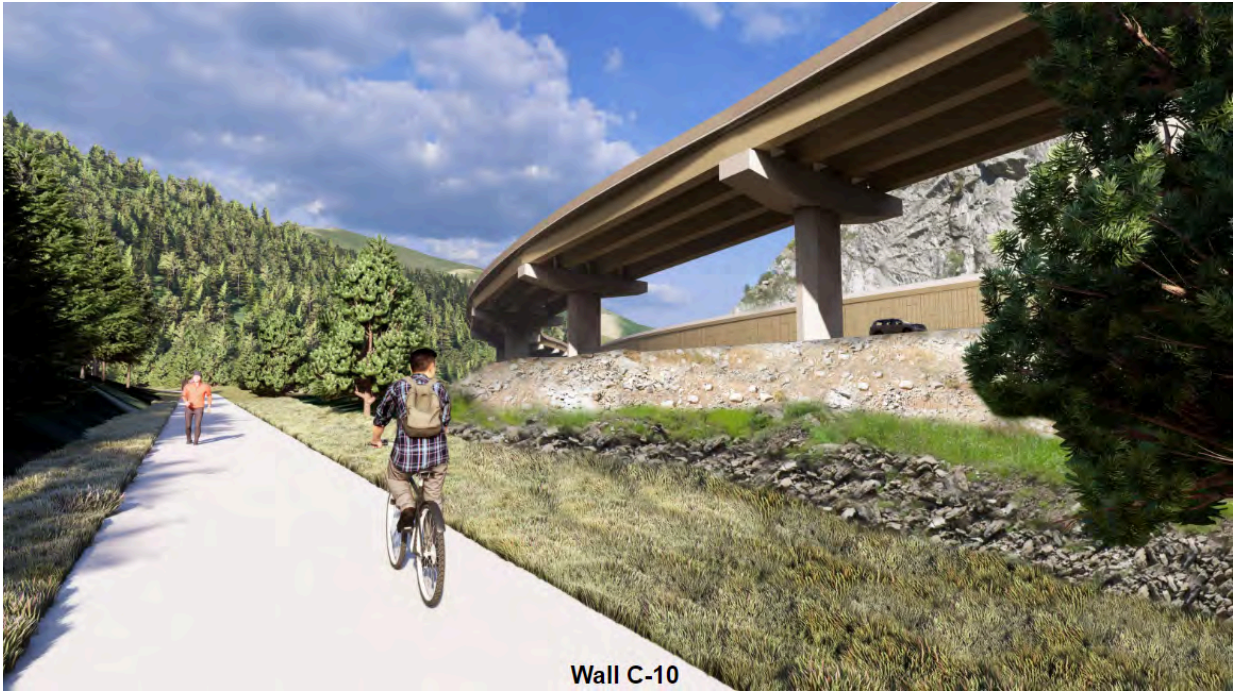
Wall C-10 seen from the Greenway Trail. The wall is seen here with 5x10 panels.
