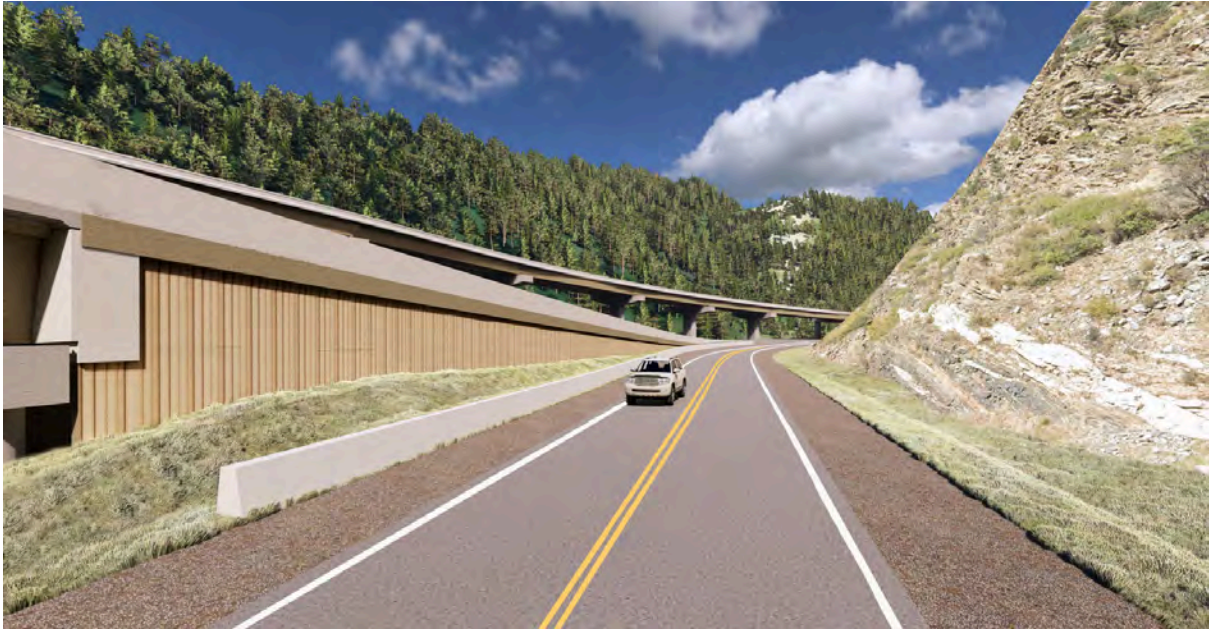
Wall C-3 seen from future US 6 looking west on the north side with Bridge M in the distance. The wall is seen here with 5x10 panels.
